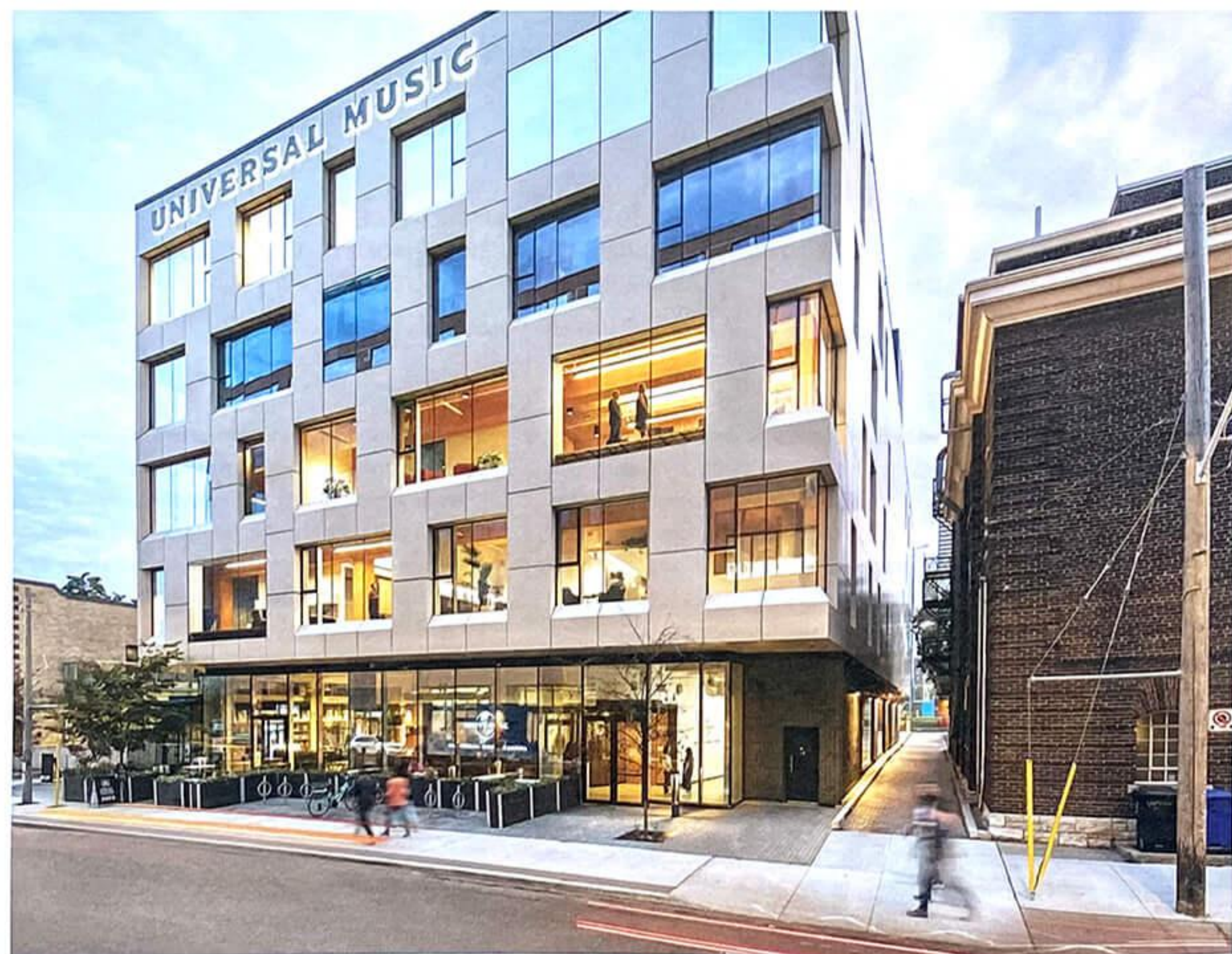
RIGHT: The HQ has a commanding street presence in Toronto's Liberty Village neighbourhood, with a ground-floor café (designed by Solid Design Creative) open to the public.
